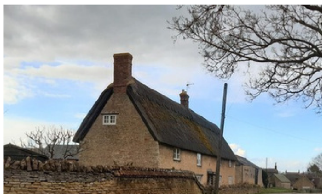
Mannings Farmhouse, coursed rubble stone walls with thatched roof
