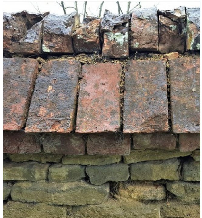
Wall detail showing coping detail to the top of the wall and the un-pointed stonework
