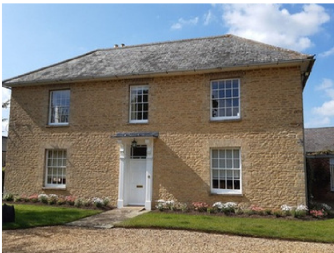
Ravenstone House relies only on symmetry and dimension to make an eloquent architectural statement. Note the brick edgings to the window, the central panel door and the hipped and shallow pitches of the Welsh slate roof
